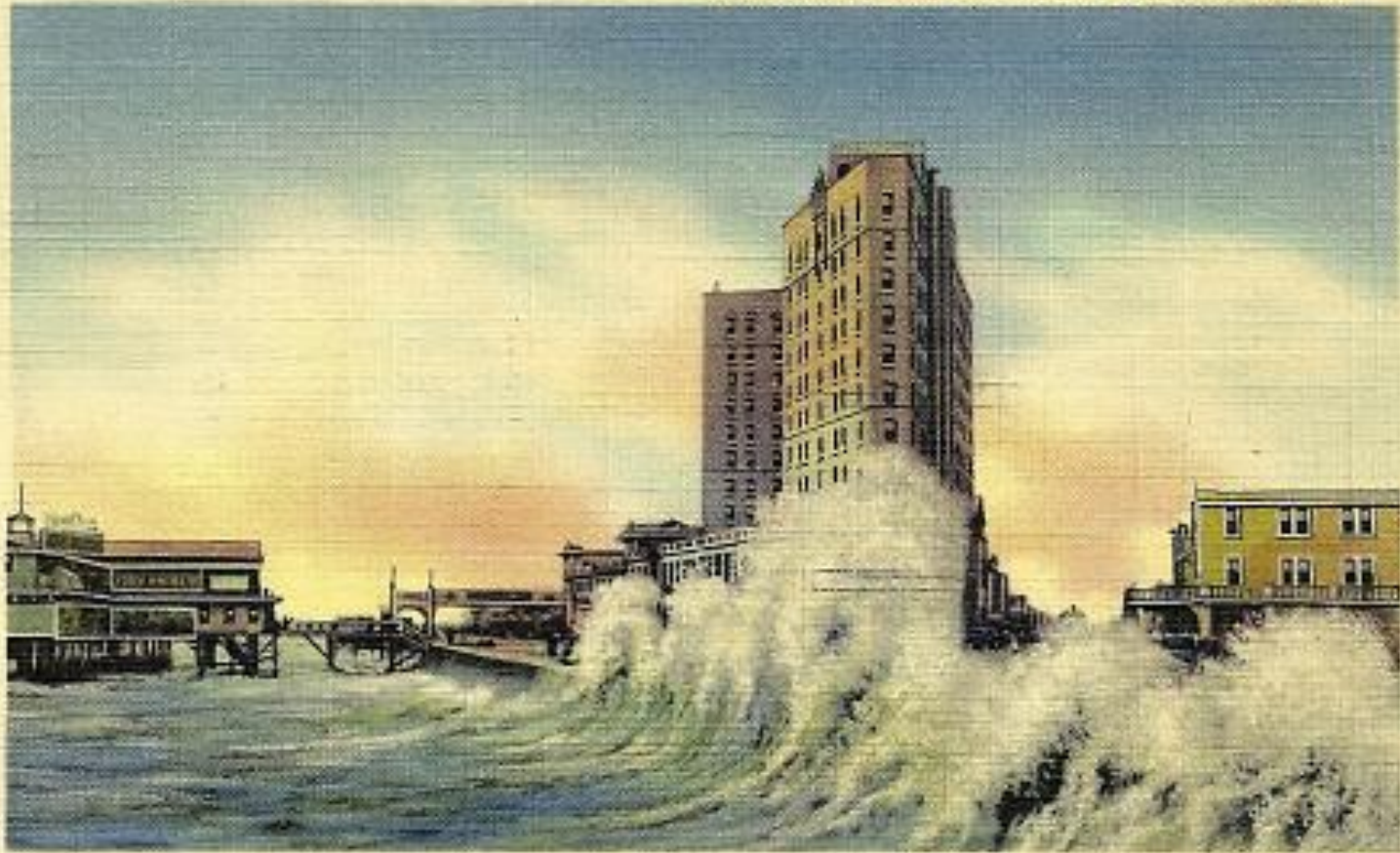
THE GREAT SEAWALL PROTECTING GALVESTON, TEXAS
